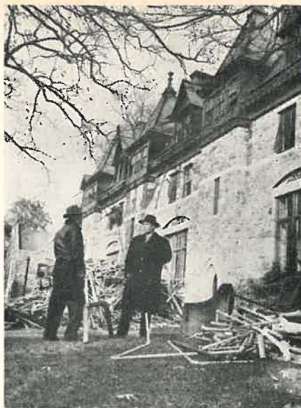
WITH ITS INSIDES ON ITS OUTSIDES St. Luke's Hall gets steam heat to replace fireplaces.
