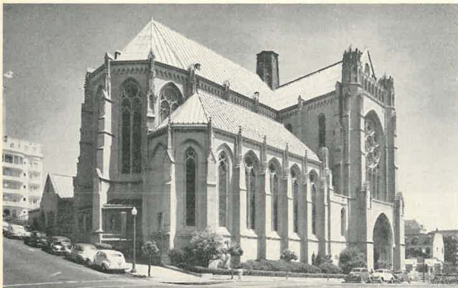
GRACE CATHEDRAL, SAN FRANCISCO: When rain and wind subsided the damage totaled $75,000.
