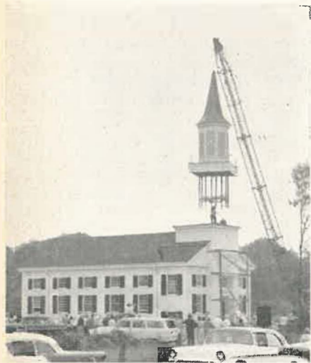
PUTTING ON THE STEEPLE was one of the last steps in building St. Ann's Church, Old Lyme, Conn.
