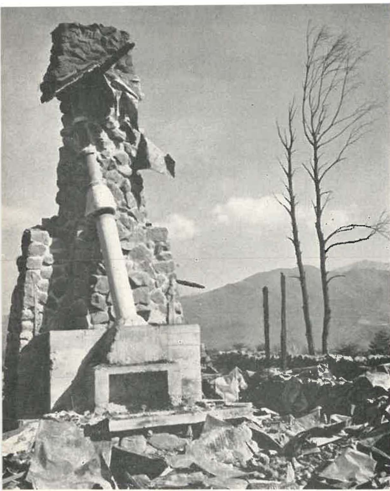
Asbes and rubble, remnants of the Seisen Ryo central lodge.
