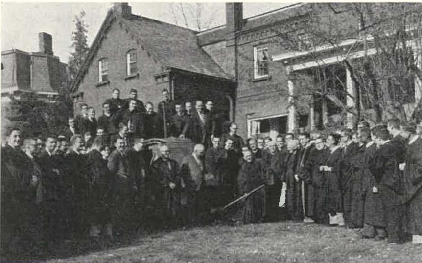
DEAN Percy Urban takes part in ground-breaking ceremonies for new library, classroom, and administration building facilities at the Berkeley Divinity School, New Haven, Conn., several weeks ago. In addition to these new facilities at the Divinity School, 102-year-old Berkeley just recently accepted three houses which belonged formerly to Yale University at New Haven.
