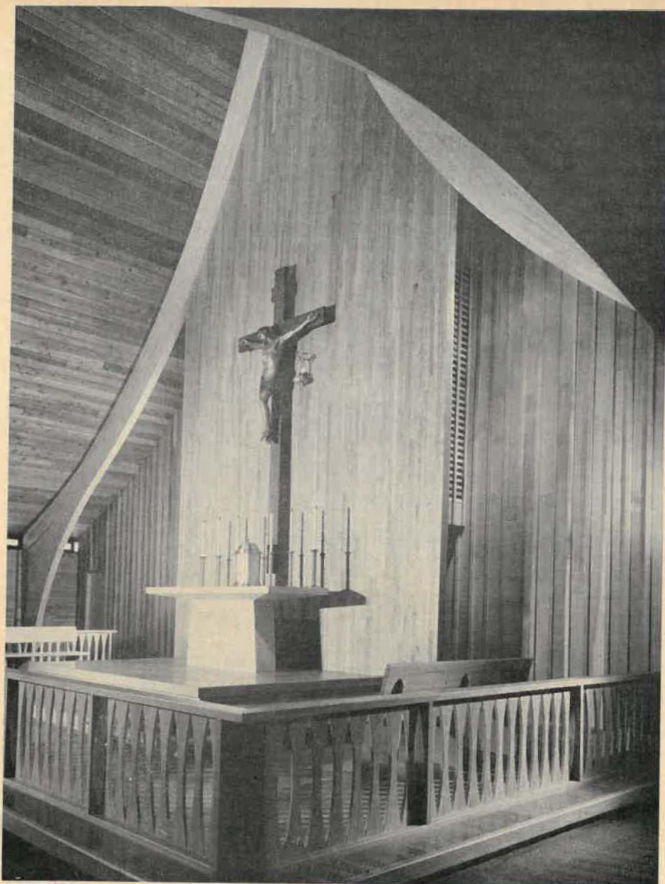
Warm colors and soaring curves in a prayerful place. The roof decking is of red cedar, unfinished so that its subtle fragrance adds to the environmental effects of the architecture. The roof seems to float above the buff brick walls and shallow windows. End walls of rough-sawn redwood echo the board and batten of the exterior gables. The polished red oak of the dorsal wall, repeated in the altar rail and chancel furnishings, forms a background for the life-size crucifix.
