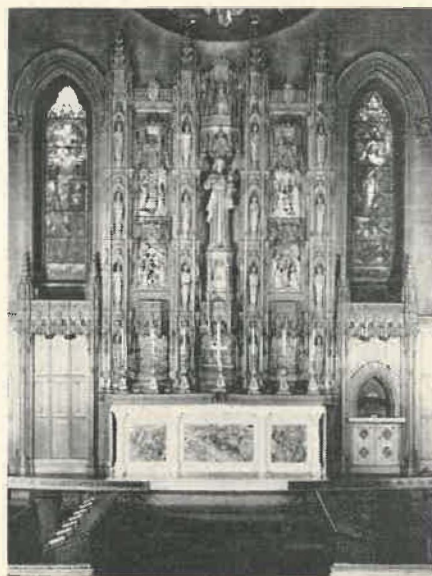
CATHEDRAL CHURCH OF ST. LUKE PORTLAND, MAINE
