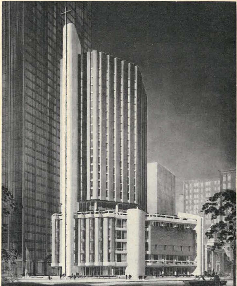
The world's largest shore center for merchant seamen, Seamen's Church Institute of New York, will be a 23-story building, to be completed by late 1967. A portion of the structure will rest on land where the old Dutch fort of Nieuw Amsterdam was situated. The five lower floors will accommodate "non-living" facilities, and the top eighteen-story tower will provide hotel accommodations for seamen. The institute, an agency of the Diocese of New York, was founded in 1834.
