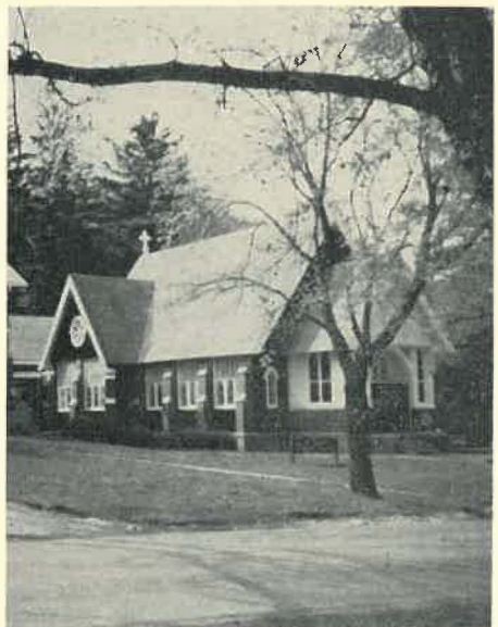
ST. LUKE'S CHURCH HOT SPRINGS, VA.
