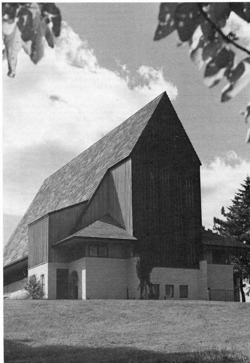
East end of the chapel at St. John Baptist School, Mendham, N.J. Chaplain is the Rev. James C. Ransom, who holds daily services at the chapel.
