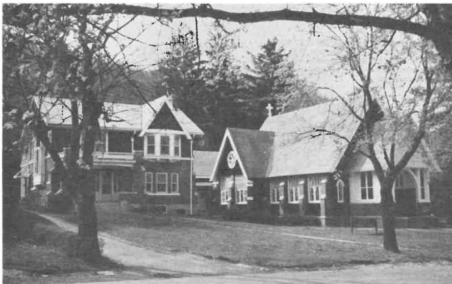
St. Luke's Church, Hot Springs, Va.
