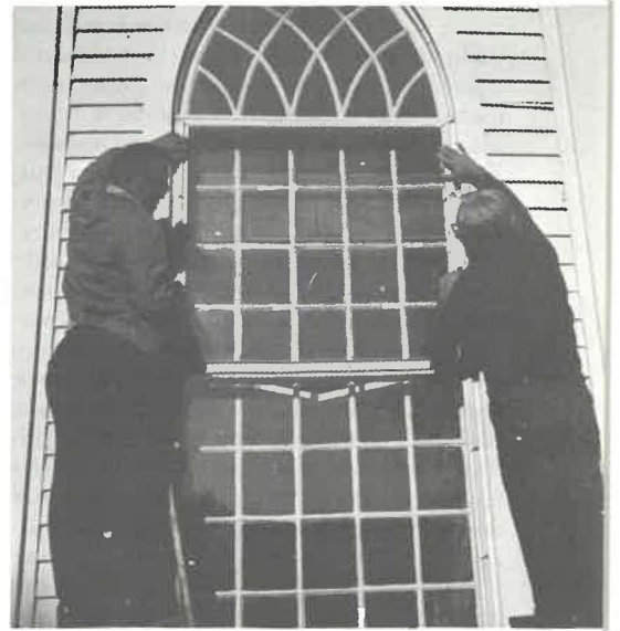
Installing storm windows at St. Mark's, New Milford.
