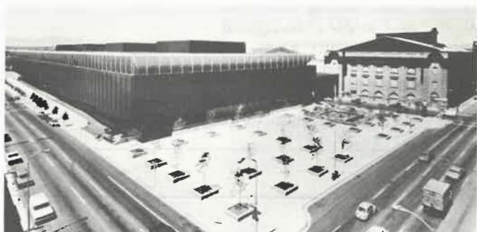
The convention site: Acoustics are inevitably a problem.
