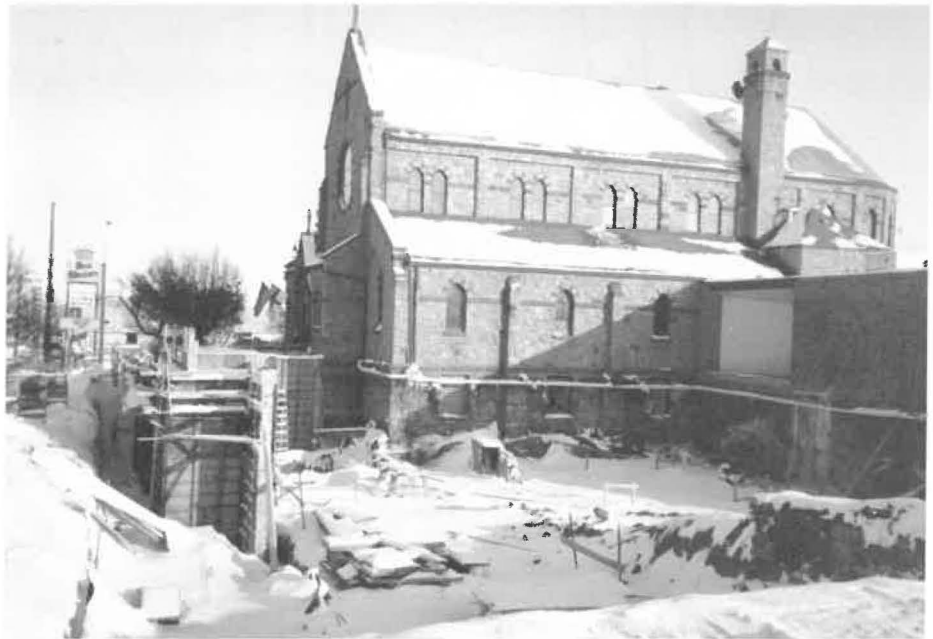
Construction is underway on the addition to Calvary Cathedral , Sioux Falls' oldest congregation, dating from 1872. Excavation began in October on the 12,000-sq. ft., two-story building addition which will cost about $1.1 million. The addition will include three new classrooms, a middle school youth center and expanded bookstore, as well as offices for the Diocese of South Dakota.
