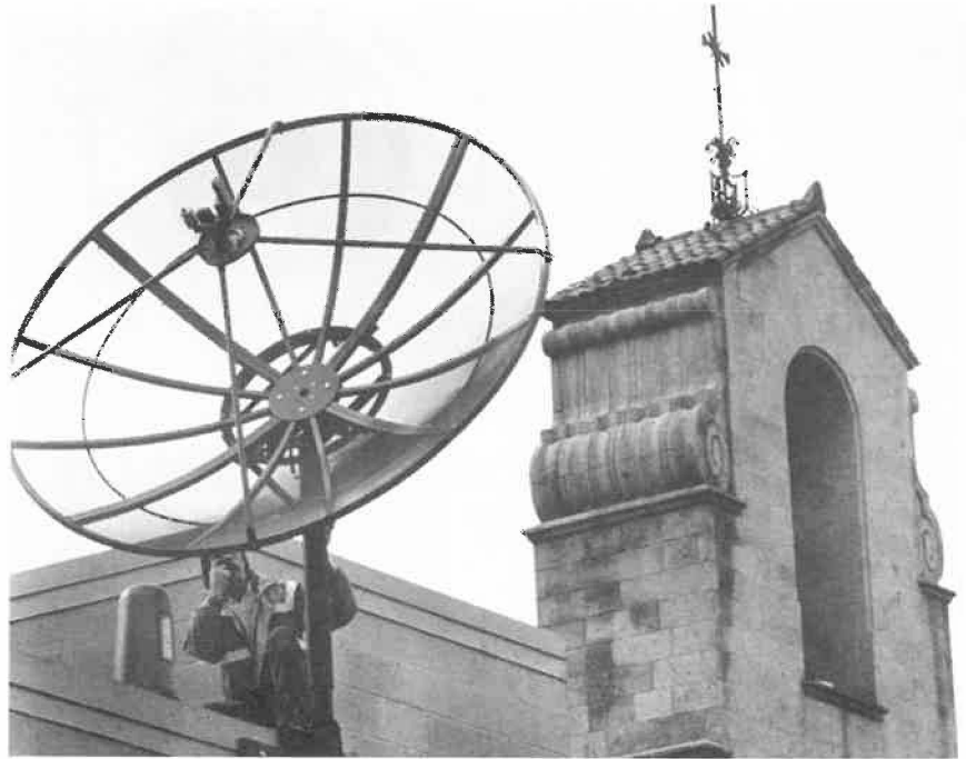
ENS photo by Nan Ross A satellite dish is installed atop Trinity Cathedral in Phoenix, Ariz., which will allow the cathedral to be linked with other sites throughout the church as part of a new national network of information and education.
