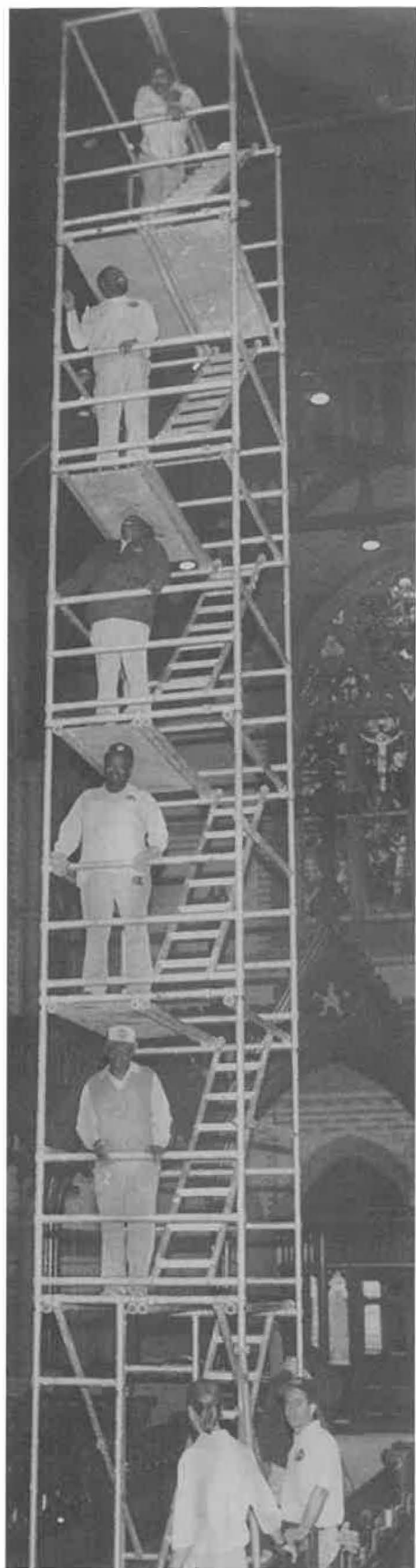
In the Chapel of the Good Shepherd at General Theological Seminary in New York City, changing a light bulb is no small task. If more than one lamp needs replacing, the task of putting up and taking down the scaffolding can take all day.
