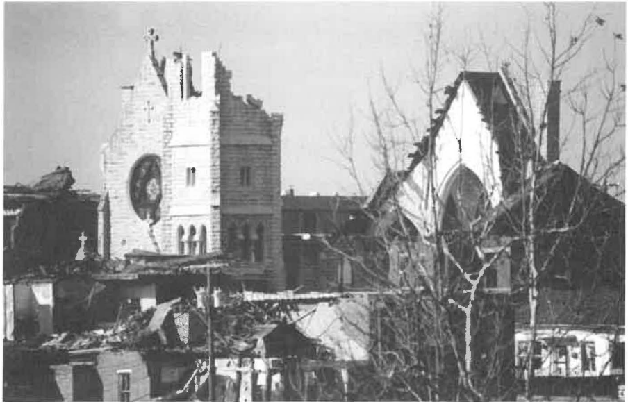
Trinity Church, Clarksville, Tenn., was destroyed by a tornado that moved through the downtown historic district Jan. 22.
